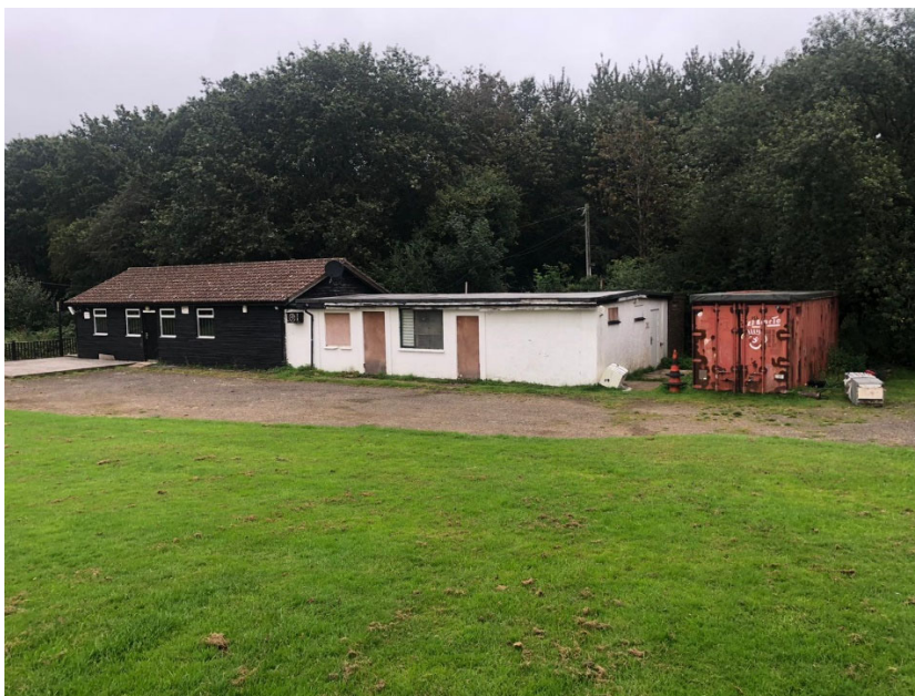
Fig. 08: Parking area in front of club house
